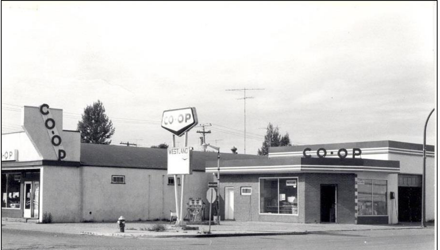
Carnduff Co-op & Gas Bar with Service Bay (c. 1965)
